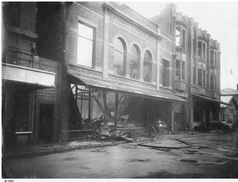
State Library of South Australia - Bentham Street, Adelaide [B 1201], Bentham Street, Adelaide, showing the business premises of the S.A. Farmers' Co-operative Union after damage by fire on 21st February 1923. The left side of the three storey building on the right is 71 yards south of Waymouth Street. The right side is 50 and a half yards south of Waymouth
